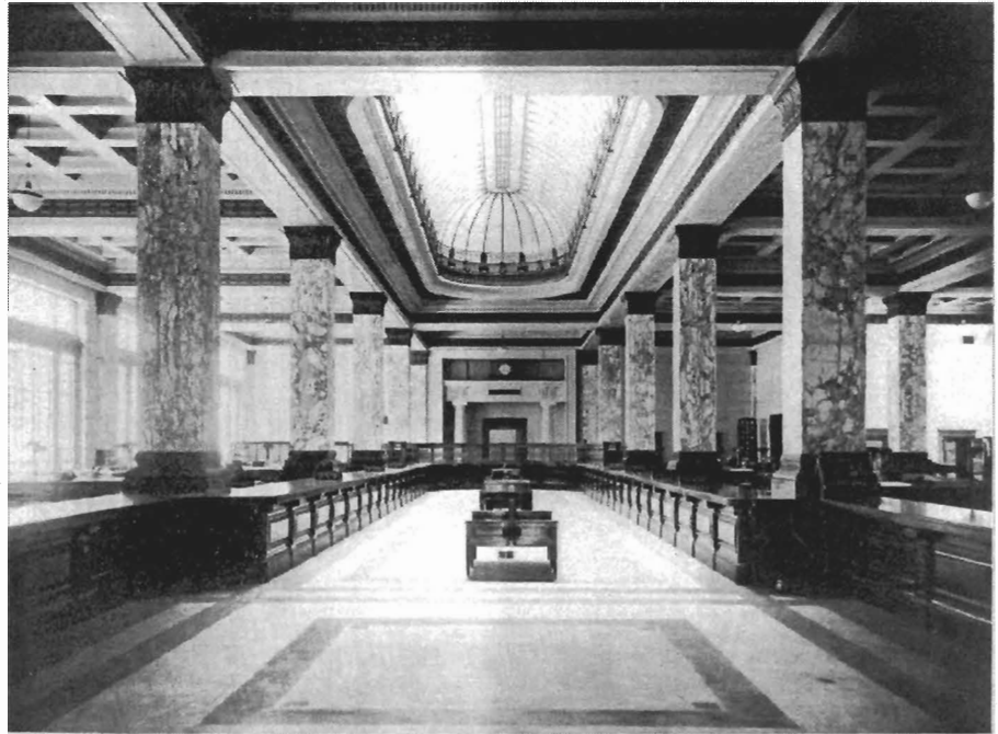
Figure 9: Hongkong Bank, Shanghai 1923: principal banking hall
