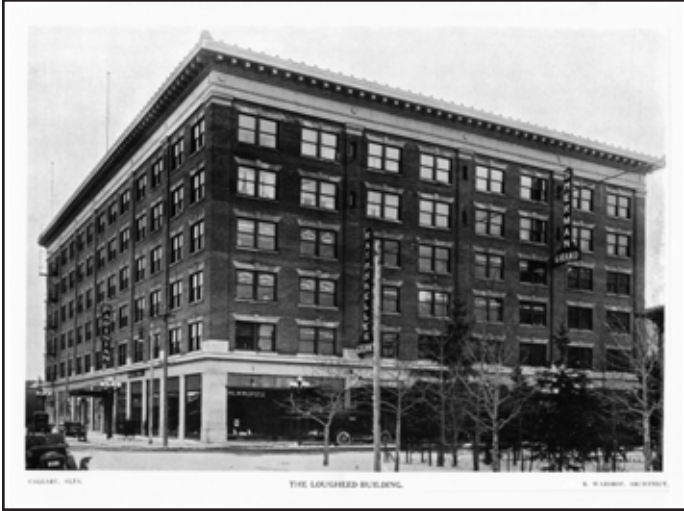
The Lougheed Building and the Sherman Grand Theatre, Calgary 1913. Photo originally published in volume 6 (October 1913) of Construction, reproduced in Donald Smith, Calgary's Grand Story, Calgary, University of Calgary Press, 2005. The history of this single building provides Smith with the opportunity of retelling a number of stories significant to the history of Alberta, among them Bible Bill, the United Farmers of Alberta and Peter Lougheed (grand son of building's original developers).
