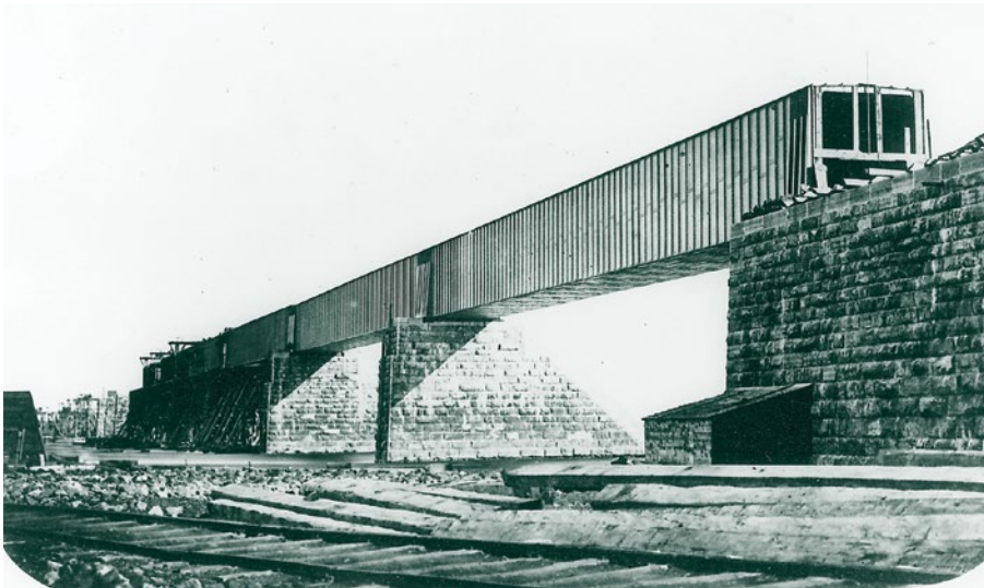
FROM BELOW NORTH ABUTMENT, VICTORIA BRIDGE, MONTREAL, QUEBEC. OCTOBER 25, 1858.
